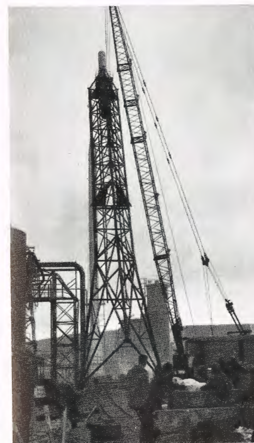
New tower. One of the most recent additions to Wilton's skyline is this 105 ft. supporting tower, comprising some 3000 separate parts, which was constructed in Wilton Works' central workshops. It is a 12½-ton triangular tubular steel tripod and is part of an extension programme to enable nearly 20,000 extra tons of nylon to be made annually by the north-east coast plants of Dyestuffs Division
